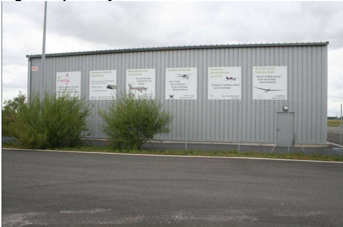
(coll Service Communication CCFL)
